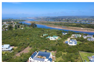
5 bedroom house in Keurbooms
