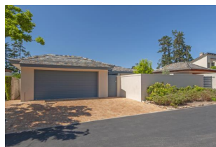
3 bedroom house in Arabella Country Estate R4,190,000
