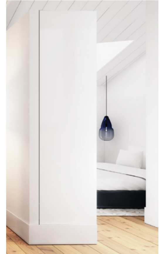
Skirting board in MDF (medium density fiberboard) lacquered in white (mate) h=25cm
