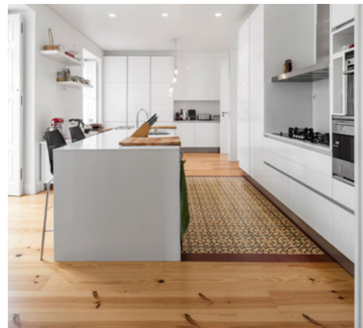
Pine floating floor (ref: Fenestevs fenwwod 220-6) & Wardrobes in MDF (medium density fiberboard) lacquered in white & hydraulic mosaic pavement in wet/sink area
